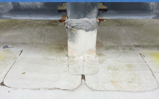
In this low spot, there were layers upon layers of patches applied to the ten-year-old roof.
