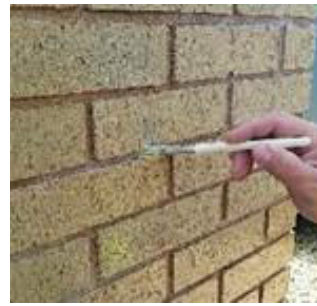
Brushing in raked mortar joints
